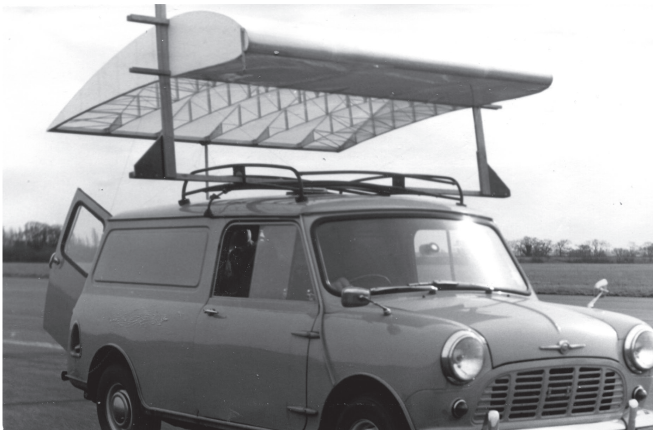
Figure 4. Wing test section mounted on vehicle.
