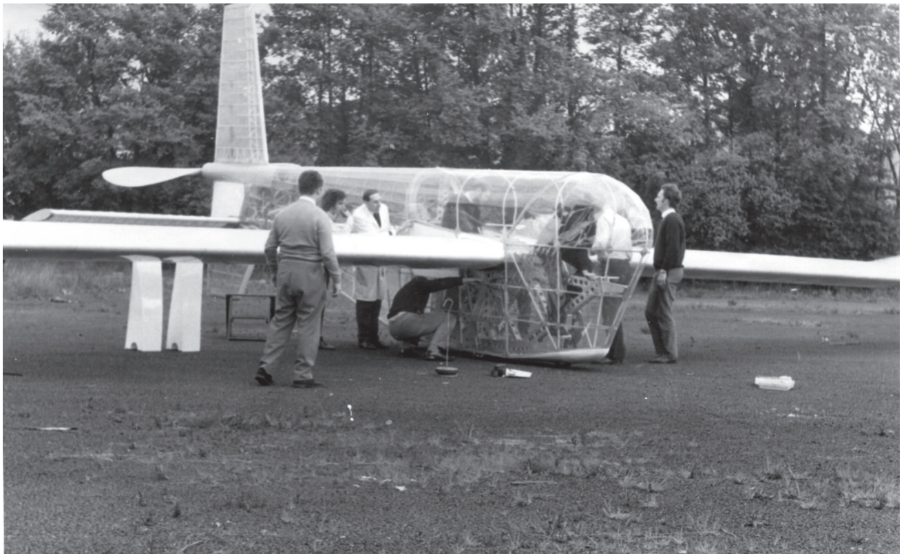
Figure 23. The transparent crew fairing and side panels are being positioned in this picture. The polystyrene trailing edge root fairings are standing on the left.
