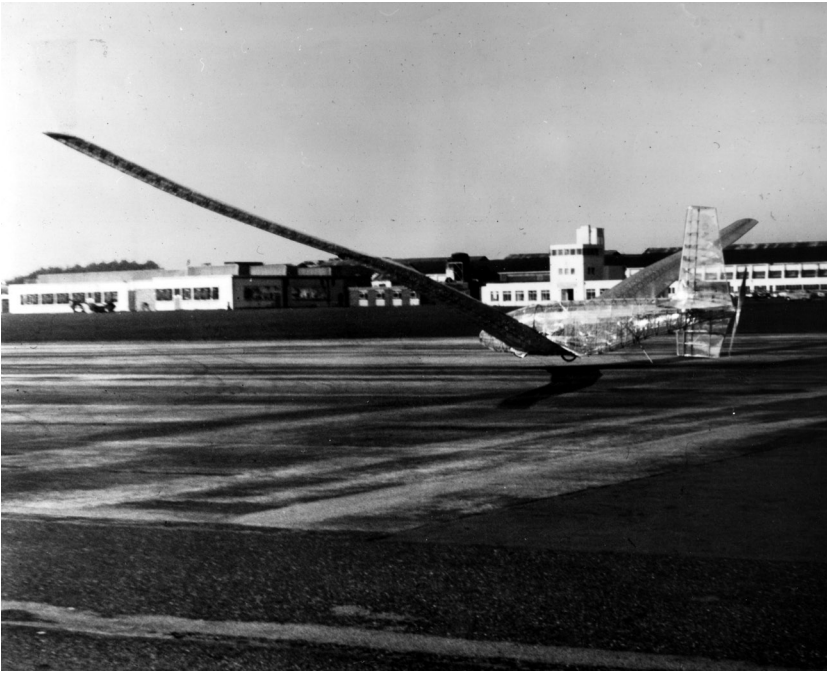
Dumbo-Mercury at Waybridge.
