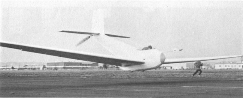
*Linnet MK II airborne above, distinguished by the cycling attitude of the pilot whereas original MK I (below) had a reclining pilot attitude. The subsequent MK III version adopts the same basic configuration of the MK II.*
