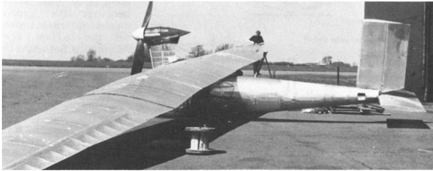
Large diameter propeller and blunt nose enclosing side-by-side propulsion/ pilots on the 'Mayfly' (centre opposite) from Southend. Rear three-quarter view at bottom shows the large tail surfaces and the Aluminised Meculon covering adopted for this, the first of the British 2-man machines.
