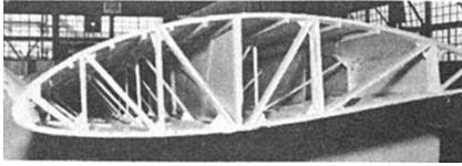
*Linnet II wing section showing structure with span-wise longerons.*
