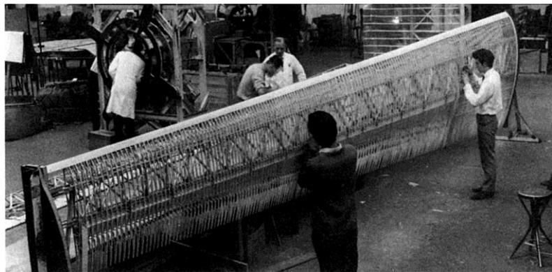
*Above top, Puffin MK 1 in flight at Hatfield with the balsa covered wings sheathed in Melinex. Above, the MK II wing under construction with fine pitch rib spacing to conserve the aerofoil. The completed MK II airframe is seen at right, with adjustable dihedral angle, and enlarged rudder giving a saw-tooth leading edge.*
