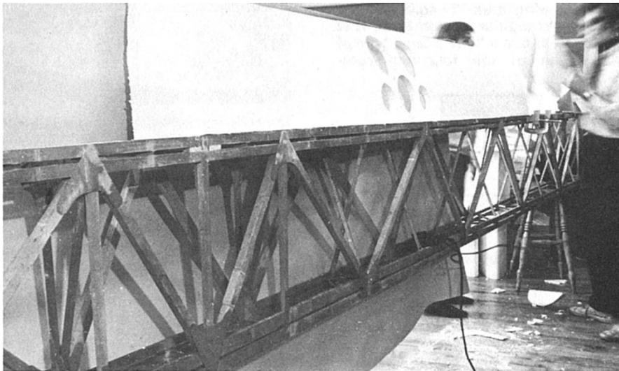
*Above: Puffin main spar unit being incorporated into Liverpool puffin wing.*
