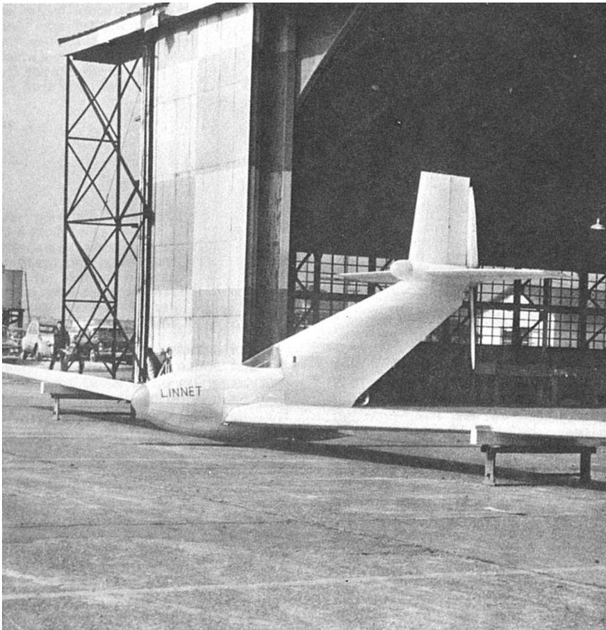
*Roll out of the Linnet Mark I which made its first flight on February 26th 1966 after basic study and construction dating back to April 1963. Wing section was NACA 63<sub>3</sub>-1218, aspect ratio 18.5. Empty weight 105 lbs. It cruised at 6 ft altitude, airspeed 17 m.p.h. Covering was Balsa on wing leading edge, otherwise styrene sheet.*
