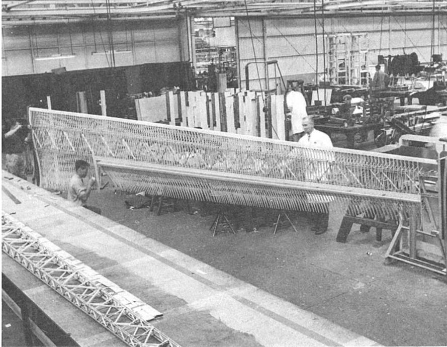
*Complexity of Puffin II wing assembly with its multiple close spaced ribs is clear in this view of the port lip panel in its jig. The Starboard panel mainspar box can be seen on the bench in the foreground. Note the large aileron area. At this stage the lip drag rudder is omitted.*
