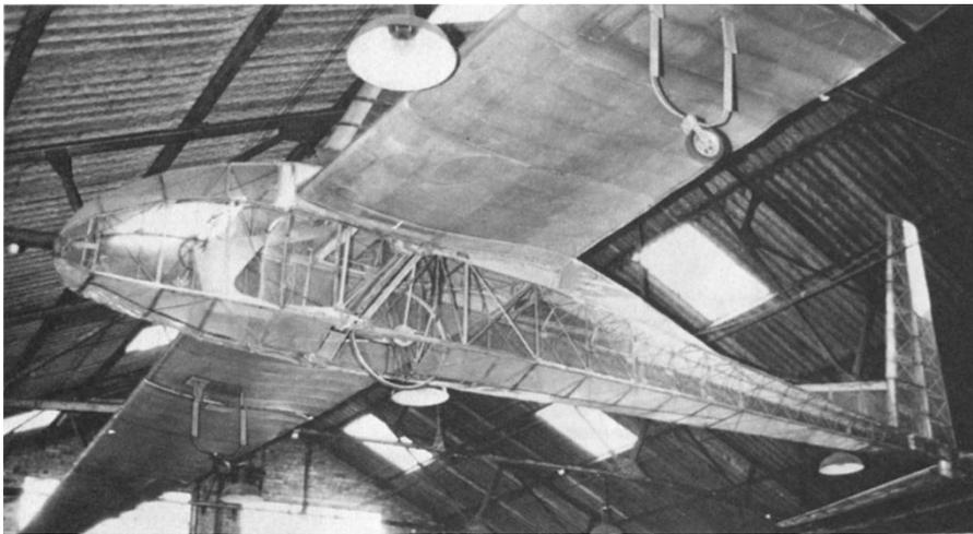
*SUMPAC is notable for its pylon mounted propeller and conventional control surfaces. A dorsal fin was added, tail area increased and light weight Melinex covering applied during progressive modifications.*
