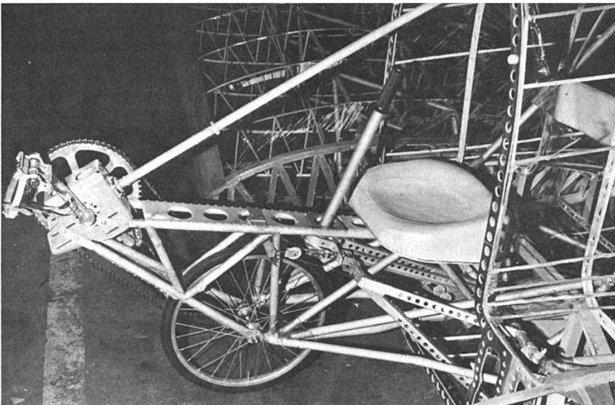
*Another view of the Weybridge aircraft reclining seat position for the pilot, also the unusual controls which can pivot entire wing panels via fulcrum under seat, for lateral control.*
