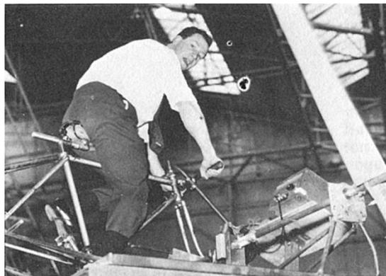
*Most man-powered Aircraft projects have a pilot test rig to assess the energy required and to check the drive mechanism. This is the unit made for training Puffin pilots at Hatfield, registering developed Horse Power as the cyclist drives the propeller.*
